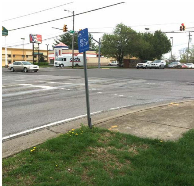
FIGURE 1 | BUS STOP WITH DEAD-END SIDEWALK (NASHVILLE) FIGURE 2 | CURB EXTENSION AND RAMP (INDIANAPOLIS)
