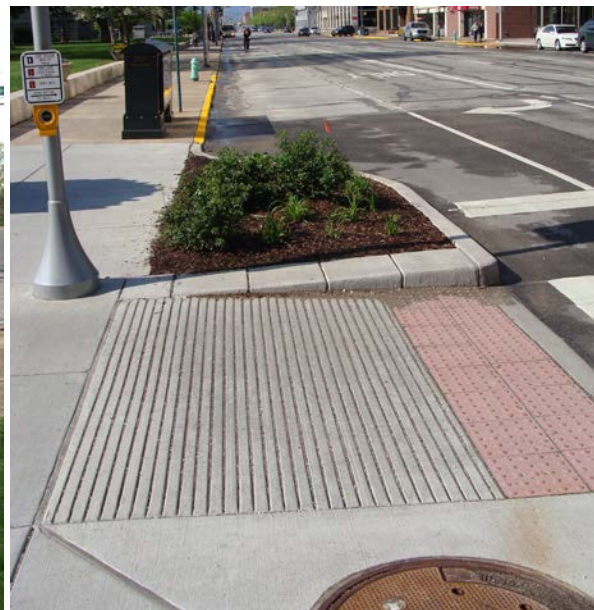
FIGURE 1 | BUS STOP WITH DEAD-END SIDEWALK (NASHVILLE) FIGURE 2 | CURB EXTENSION AND RAMP (INDIANAPOLIS)
