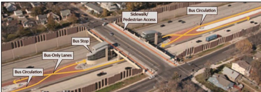
This station was constructed within a narrow median and uses center platforms to reduce the station width. However, most buses only have doors on the right side, which is the wrong side for typical center platform operations. To deal with this issue, once within the bus-only area, buses cross over to the left side so that they can board and alight passengers through their right-side doors.
